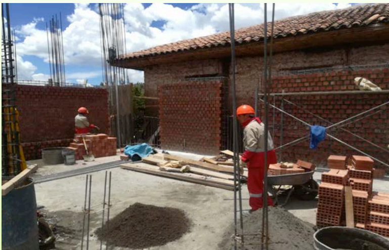
New Cusco school under construction
