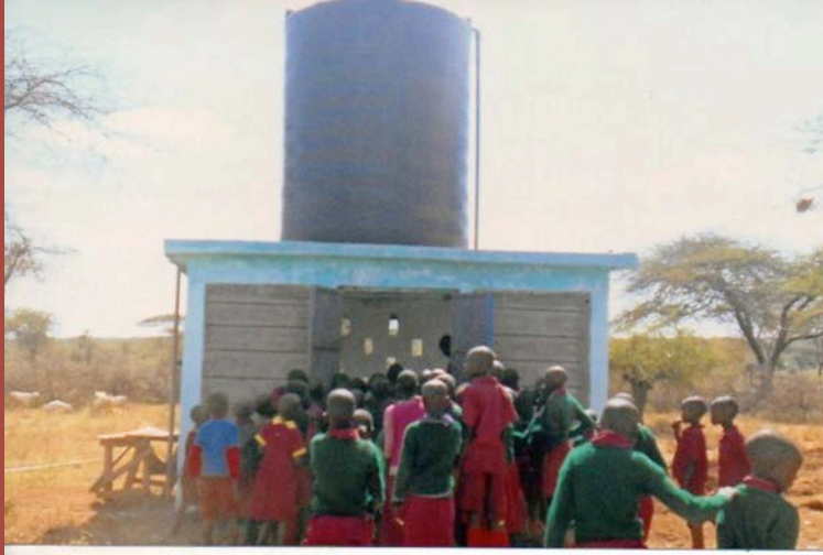
The water well at the Masai Mara School - supplying water to the children
